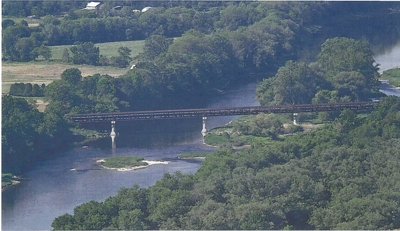
A bridge carries municipal services across the Grand River from an area near Brant Park (at left) to the city's northwest industrial area.
