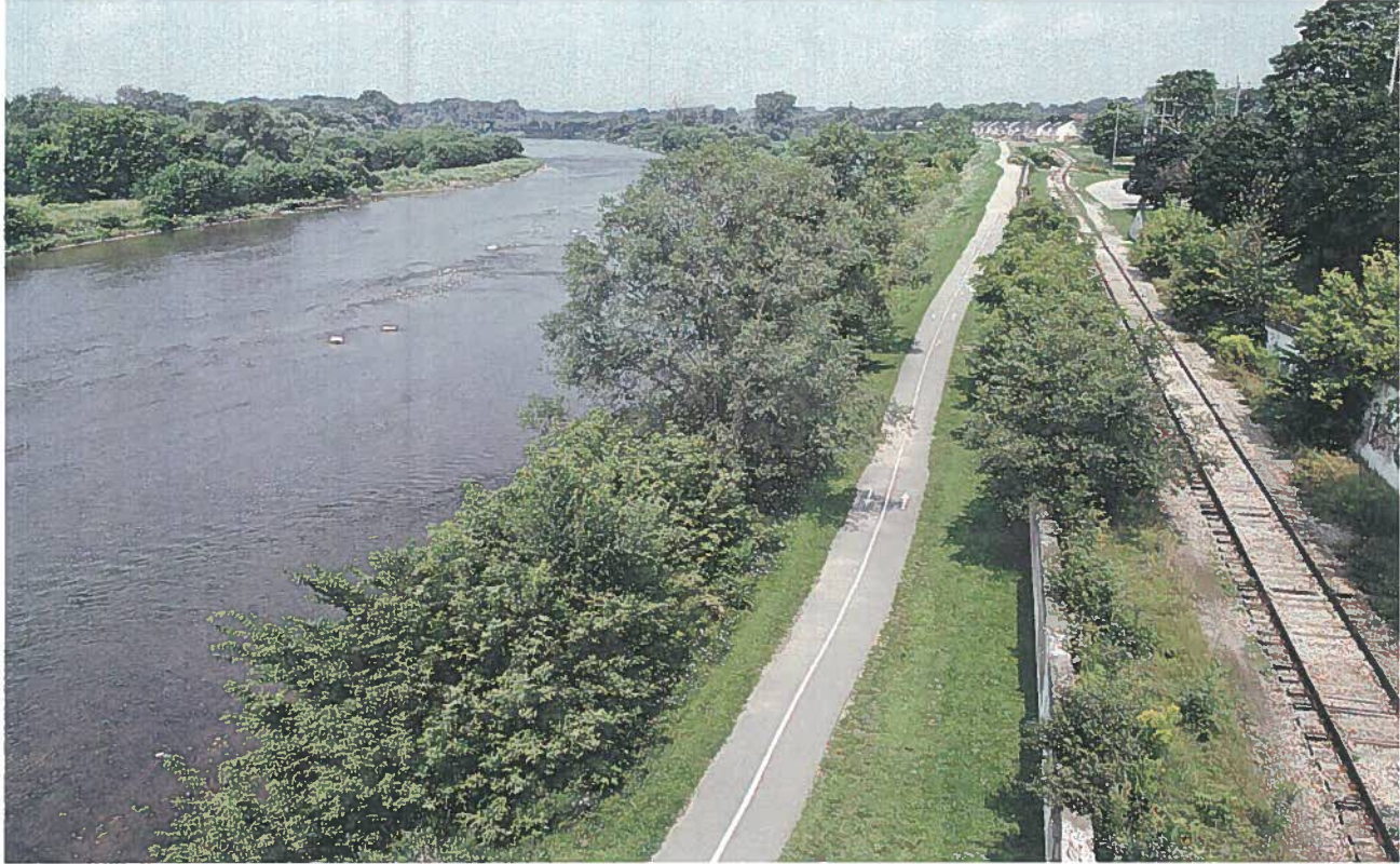
A view from Lorne Bridge of the paved trail atop the dyke, and the CNR tracks in Holmedale.
